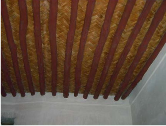
Building Construction. Fig. 7 Roof structure (Dubai) beams, mats, and mud as topping (photo by the author).
